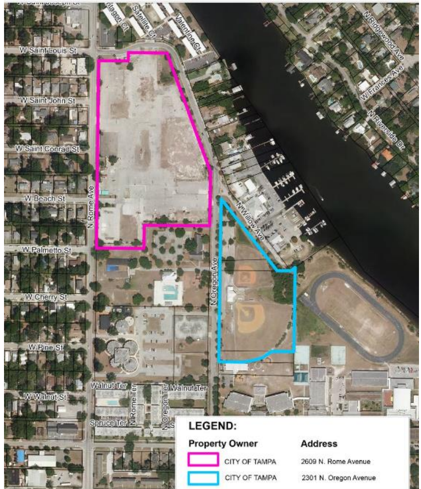
West River area the city of Tampa wants to develop
